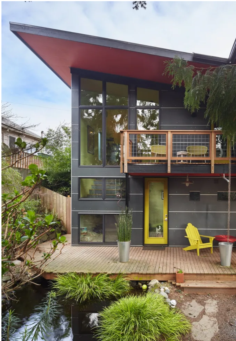
THE CLUBHOUSE. With its soaring butterfly roof, extra-wide red eaves and sunshine-yellow back entrance, this renovated home (now with a new second floor) looks through a colorful lens at a Phinney Ridge backyard filled with greenery galore and a waterfall that obscures street noise. (Benjamin Benschneider / The Seattle Times, 2016) Less ^
