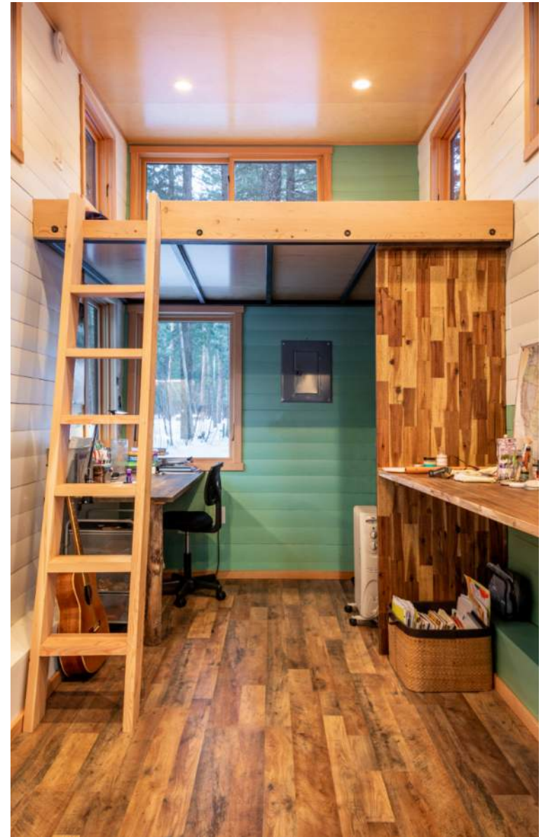
The walls are covered in six-inch pine shiplap siding painted in a creamy white and soothing green. The ceilings are clad in finished birch, and the spaces are trimmed in D-grade fir to keep costs down.
