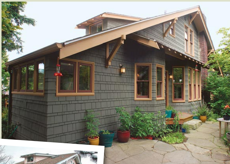
A new back door between bays. The breakfast-nook bay takes its shape and detailing from the bay in the dining room to its right. The new door is between them, sheltered by an extension of the existing shed roof. Photos taken at D on floor plan.
