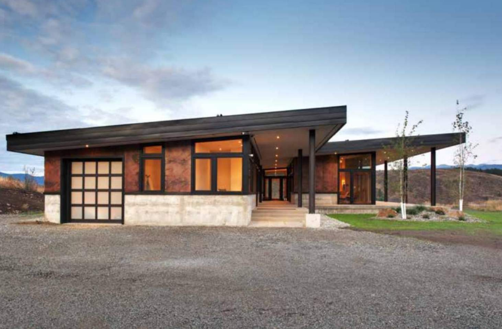
The home, designed by architect Tim Hammer of Seattle-based CAST Architecture, has an exterior made rusted steel and concrete.
