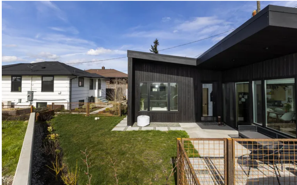
1 of 2 | Chris Cloud and his partner Adi Braun built their backyard ADU cottage, right, seen Monday, March 6, 2023 on Beacon Hill in Seattle, which they live in while renting out their main house, at left.(Ken Lambert / The Seattle Times)
