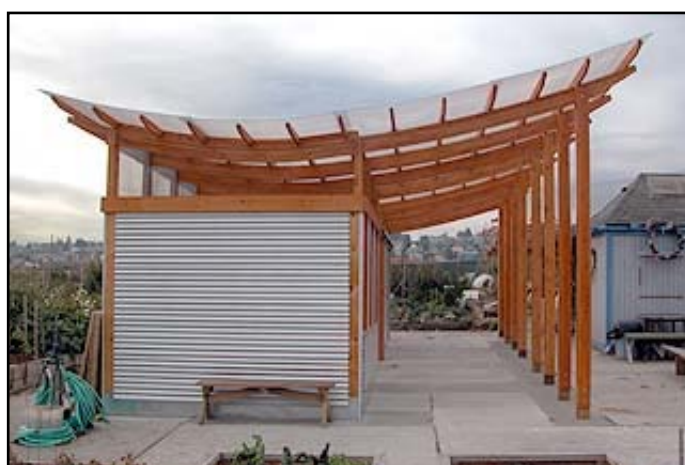
CAST's Interbay P-Patch was a pro bono project. The concave roof catches water for a portion of the garden.
