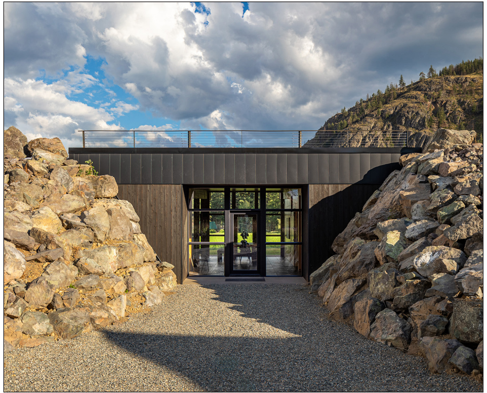
The home's main entry, shown here, is designed to look as if "emerging" from the landscape.
