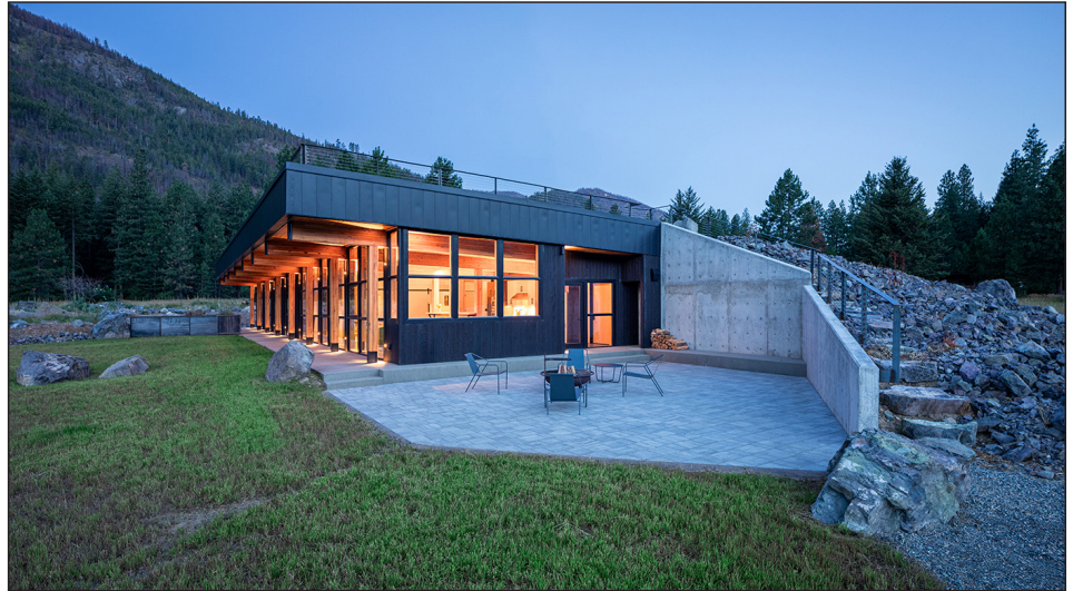
The home is built into a meadow slope and has an accessible bermed roof.
