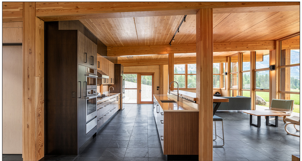
The structure is built with CLT, which is exposed on the interior.
